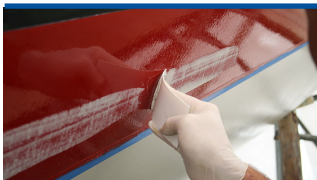
Fill along boottop
